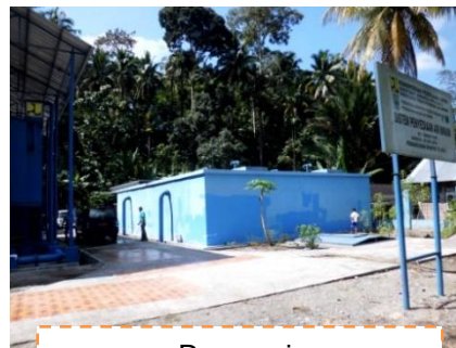
Reservoir Air Kelok
